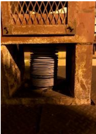
Molded Bellows in Coal Fired Energy Plant
